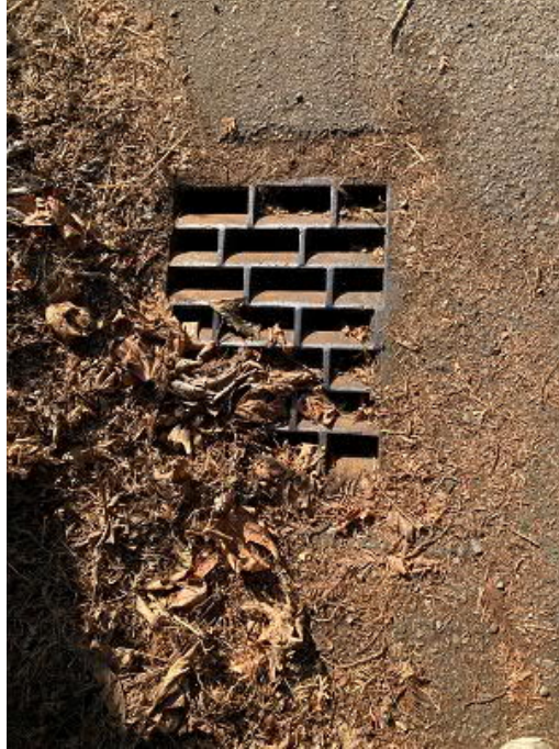
Picture 11 ROW in front of 3640 73 rd Avenue SE (south)
