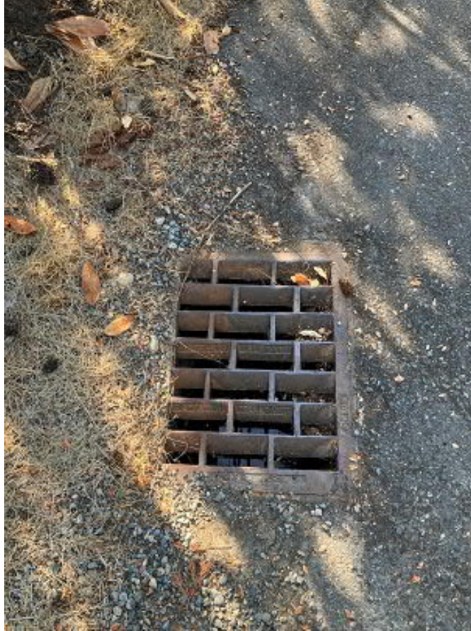
Picture 6 ROW in front of 7337 SE 36 th Street Water discharges toward the south in this 12" concrete pipe. CBs are on the east side of the street on this block.
